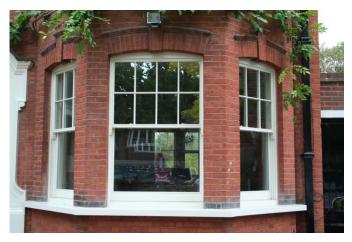
Modern tapes & adhesives securely bond the bars to both faces of the glass. The depth of the unit is only visible when viewed up close.
