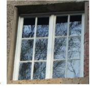
cylinder glass used in the lower section.
